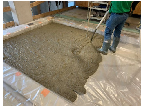
Figure 3. Application of the EPS thermal layer
