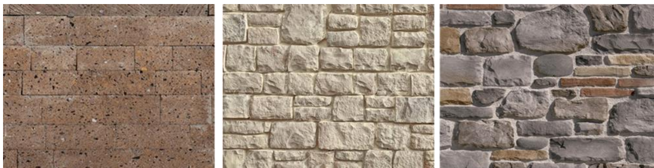
Figure 1: Structural natural stone masonry vertical partitions; Etruscan tuff/claystone masonry wall, limestone masonry wall and huddled/mixed stones wall.
