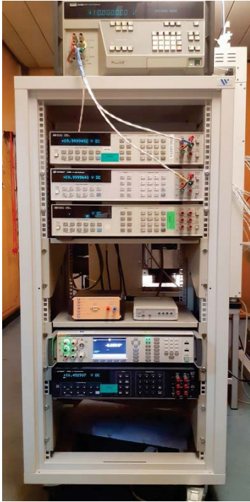
Fig. 3. The whole apparatus has been built inside a rack and, for clarity reasons, all the devices are shown together. In real measurement situations, to reduce both electrical and thermal noise, only the operative units are connected and powered. The side shields of the rack are normally removed to help with normal thermal cooling of the instruments
