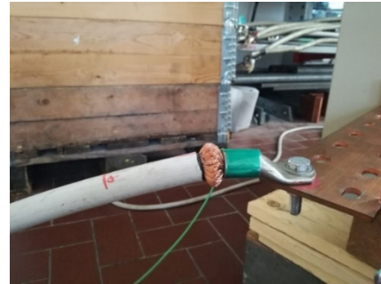
Fig.14. Swelling of the bare cable area.
