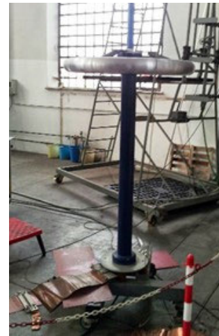
Fig. 2. HAEFELY R600 damped capacitive divider.
