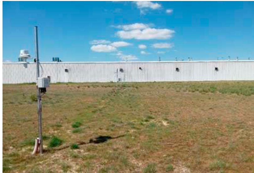
Figure 3. View of the wall of the building.
