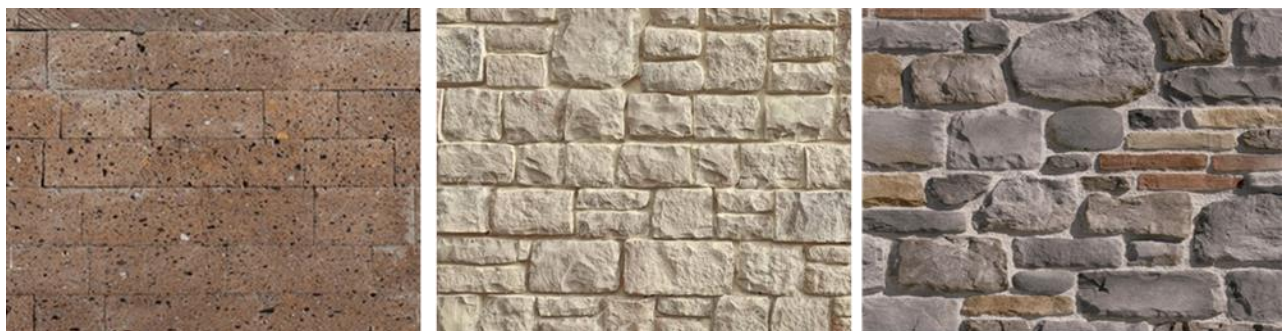
Figure 1: Structural natural stone masonry vertical partitions; Etruscan tuff/claystone masonry wall, limestone masonry wall and huddled/mixed stones wall.
