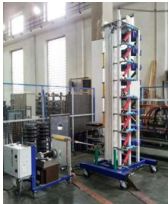
Fig. 2. LATFC's Haefely Impulse generator.
